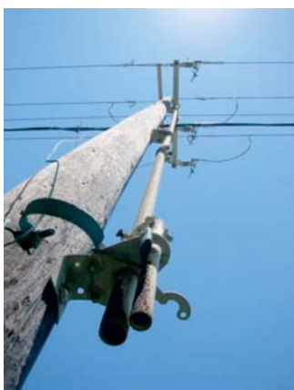
Manual switch on electricity pole
