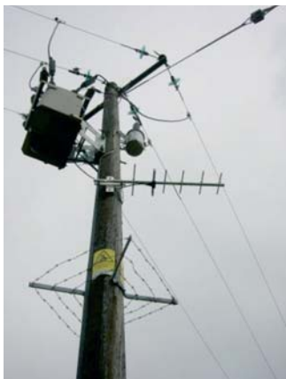
Radio-controlled switch on electricity pole-top
