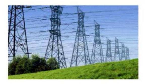
One gas pipeline (Ø 1,20 m) transports as much energy as eight power pylons (3 GW each).
